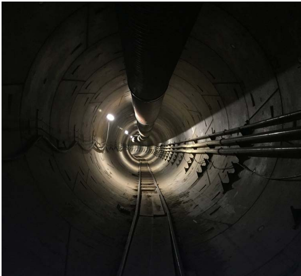
Photograph provided by The Boring Company: Tunnel
